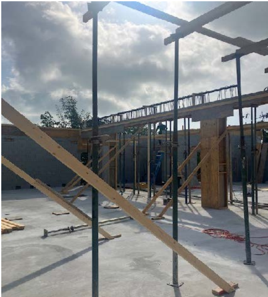
3rd Floor Beams Being Tied into Columns
