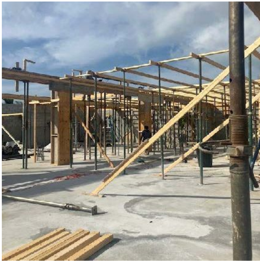
3rd Floor Beams Being Tied into Columns
